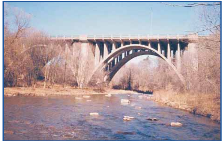
16 Mile Creek Bridge - Oakville
